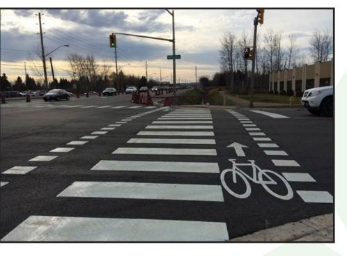
A combined crossride is comprised of "elephant's feet" markings, with "zebra stripe" markings inside. Pedestrians are intended to make use of the central area, and cyclists to use the outer parts.
