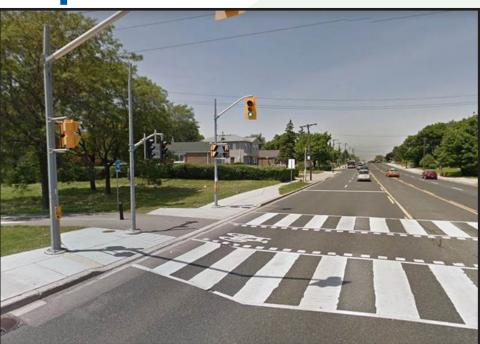
The separated crossride consists of "elephant's feed" markings in the centre, surrounded by "zebra stripe" markings on both sides. In this configuration, cyclists are intended to use the centre part, and pedestrians the outside.
